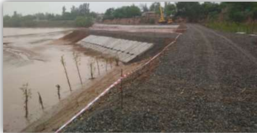
Site condition during construction
